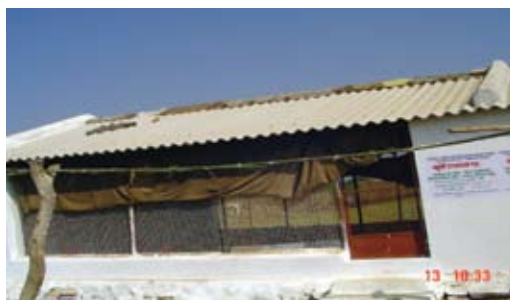
Fig. 6: AC Sheet Roof Shed
