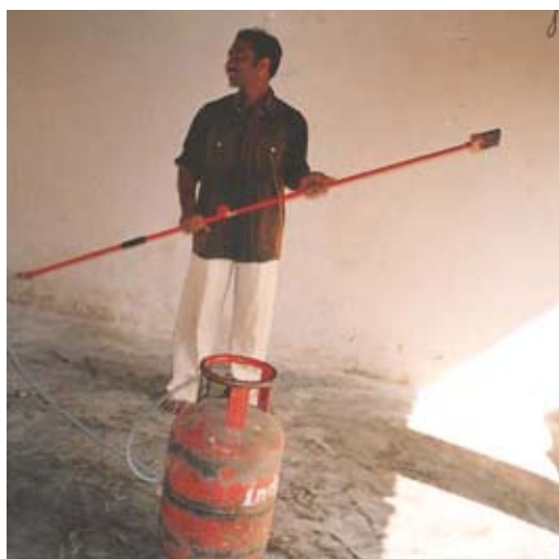
Fig. 15: Use of flame gun for cleaning
